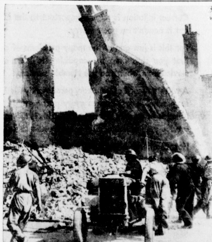
CAUTION IN CANTERBURY—Demolition of still standing brick walls and chimneys in ruins continues in Canterbury, England, in wake of devastating air raid launched by Nazis in Cologne reprisal.
