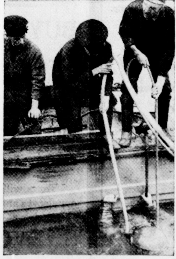
GOING DOWN FOR HULL INSPECTION.
