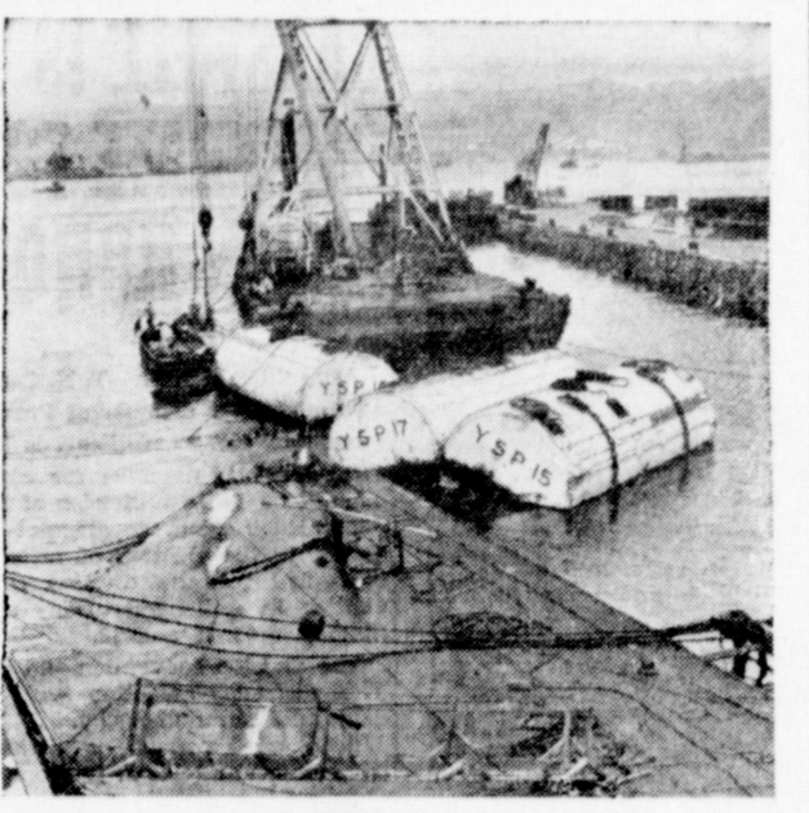
SALVAGE AT PEARL HARBOR—Salvage work continues on the hulks of ships sunk in Japanese assault on U.S. Naval Base at Pearl Harbor. Work progresses on minelayer Oglala (foreground).
