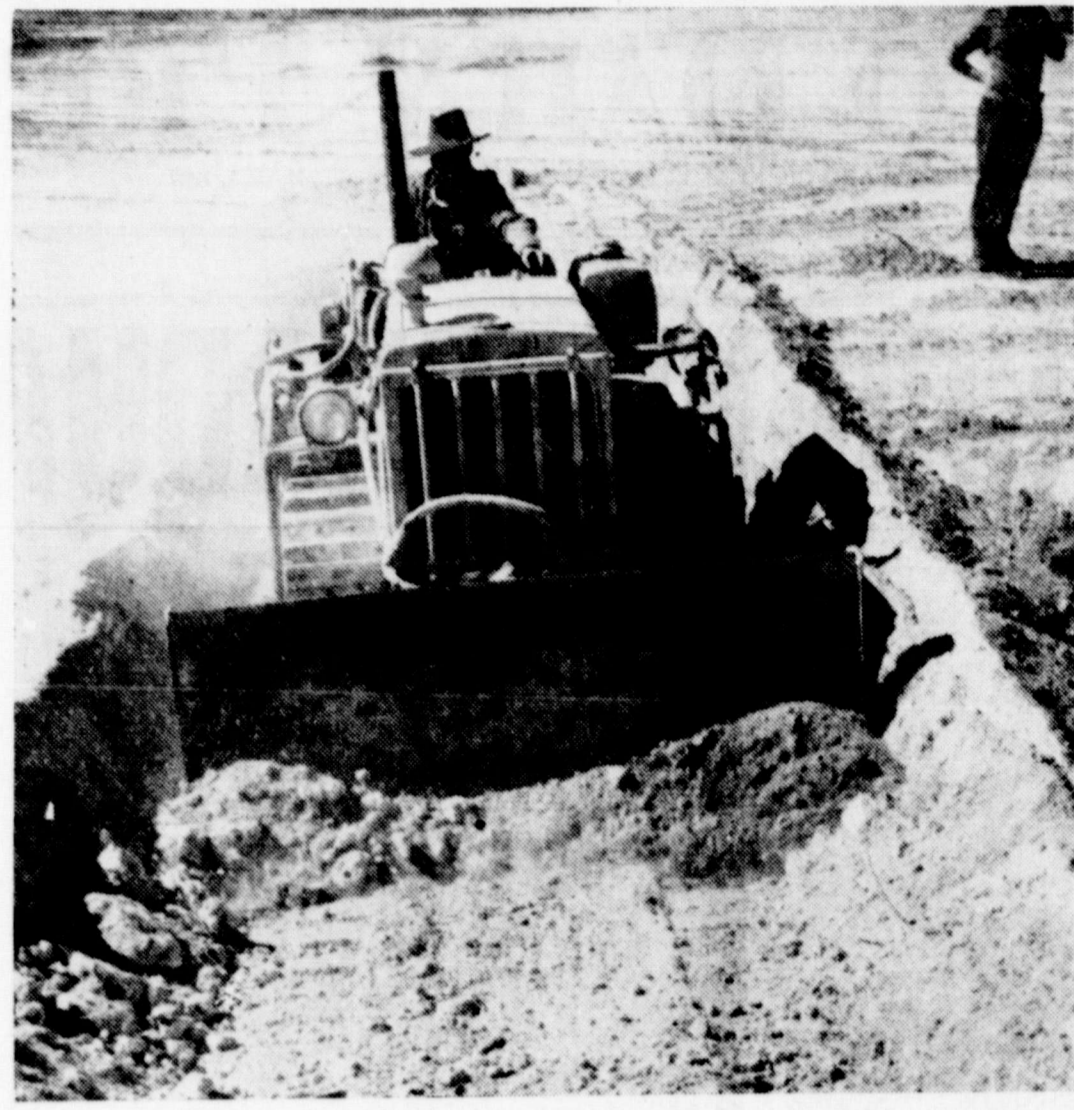
TRULY A MACHINE WAR—British forces in the Western Desert are spared many an aching back as this tractor performs the manual labor involved in "digging in" a column of supply trucks as a protection against strafing enemy planes. Machine is a "bull-dozer."
