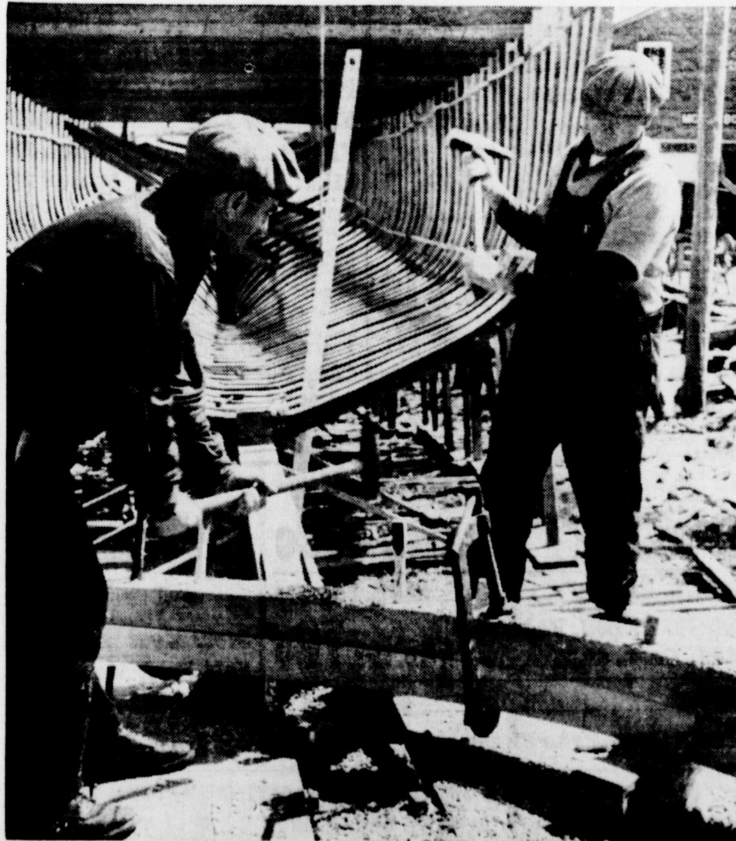
MOULDING WOODEN RIBS FOR HULL. PEGS SUPPLANT NAILS.
