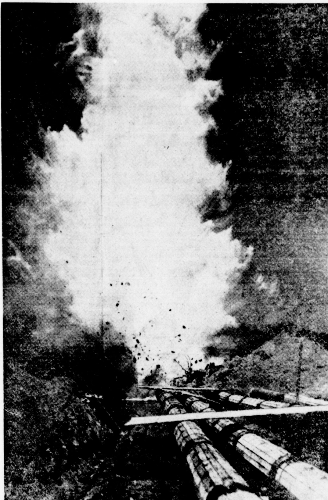
A FRIENDLY BLAST—There was no enemy weapon of war at the other end of this earth shaking blast "somewhere in the Carolinas." To the contrary, blast is clearing rock obstacles in path of oil pipe lines between Louisiana and North Carolina for Eastern defense plant.
