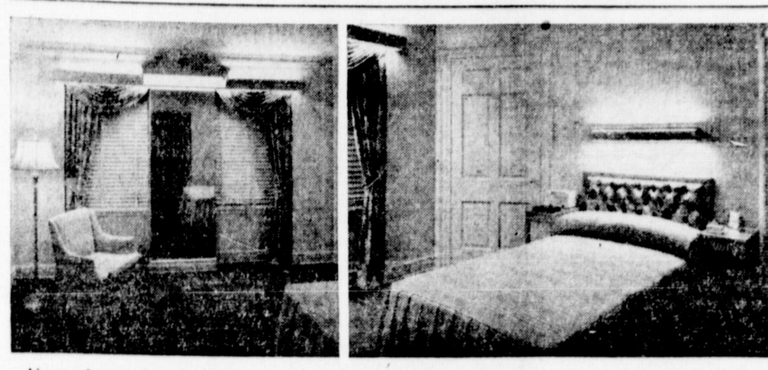
Above mirror and head of bed, streamlined fluorescent lamps produce a wealth of cool lighting for make-up and reading. Note, too, the floor lamp next the chair. This portable uses a 3-light filament lamp designed to give milady enough light for almost any sewing or reading task.
