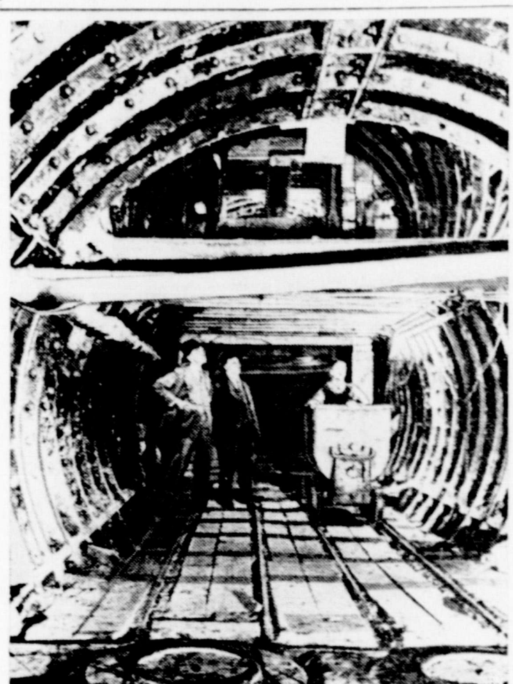
Britain is busy this summer building shelters for air raids expected in the fall, and is making best use of her space with double-deckers. Tube-shaped tunnels deep in the ground are divided into two stories to accommodate thousands of people. Banks will line walls.
