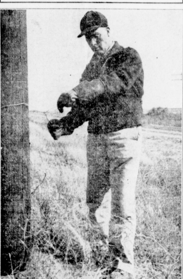
Lineman J. B. Handley of Childress shows how ordinary fence wire was used for climbing hooks in emergency that won national honors.
