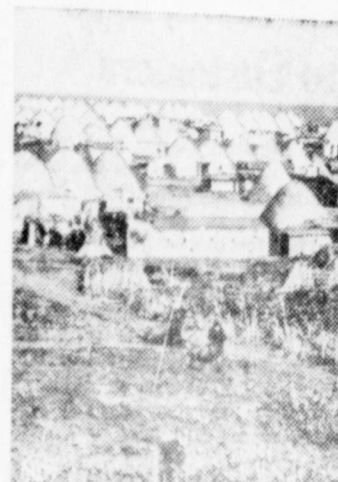
Typical Syrian town features domes for roofs. Construction helps make interiors livable despite intense heat.
