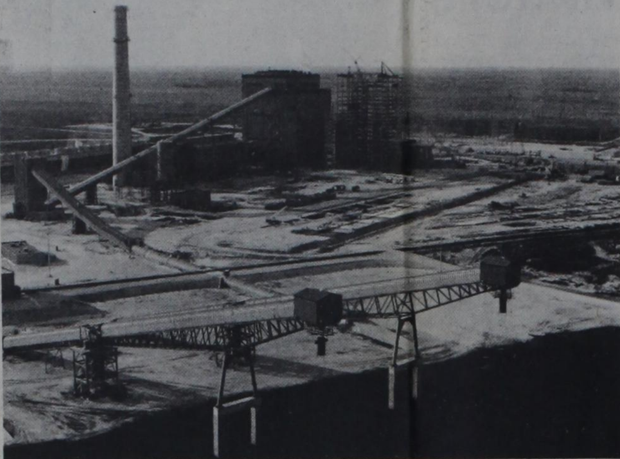
TOLK STATION —Low-sulphur coal, stockpiled in the foreground, powers Southwestern Public Service Co.'s new Tolk Station Unit No. 1. The coal is moved by conveyors into a crusher house and pulverizers which grind it as fine as talcum powder. It's burned in a boiler housed in the giant finished building [center]. The steel-framed structure next to the finished building will house Unit 2, scheduled for completion in 1985. At left of the finished building is the baghouse, which cleans flue gases on their way to the chimney stack. Public open house at the new plant will be held Saturday and Sunday. [SPS Photo]
