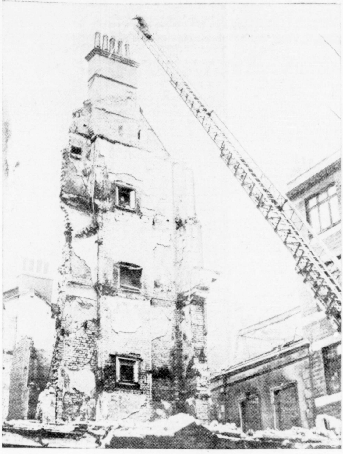
Spectacular picture illustrates one of tough jobs left for Londoners after the bombers have gone. A demolition worker goes way up there on a giant crane to fix steel cables to the wall of what was an office building before remains are tumbled down.
