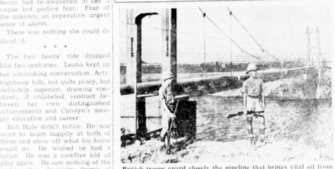
British troops guard closely the pipeline that brings vital oil from Iraq fields to warships and machines in the Mediterranean. This view shows the pipeline as it crosses the River Kishon, near its terminus in Haifa, Palestine port.
