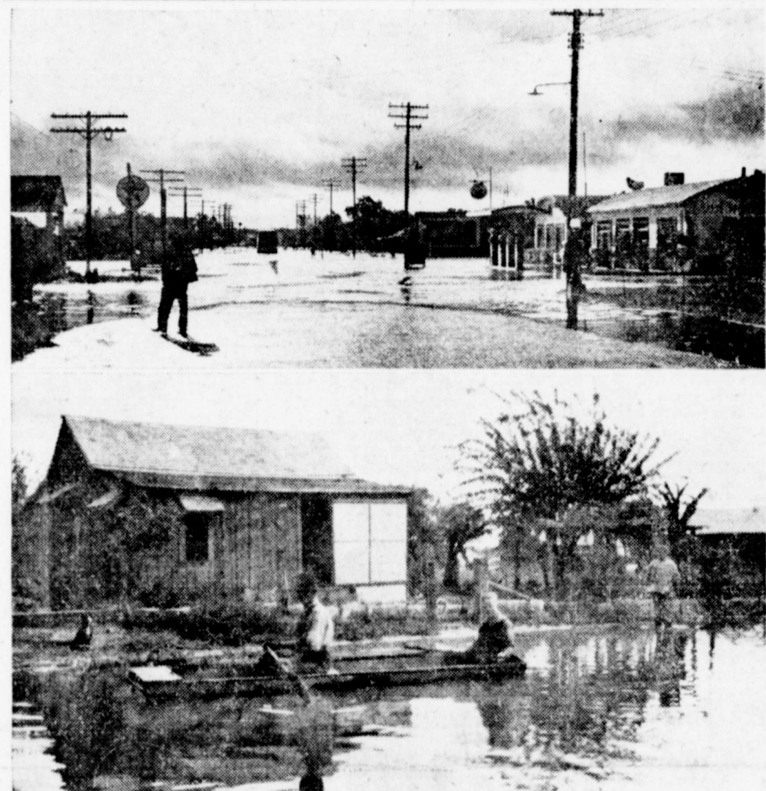
Water washes over highway 80 on eastern edge of Eastland, Texas (top photo) after heavy rains brought creeks out of their banks. In the bottom photo Joseph White arrives home via boat as flood waters surround his Brownwood, Texas, home and rise to within few blocks of county court house. (NEA Photo)
