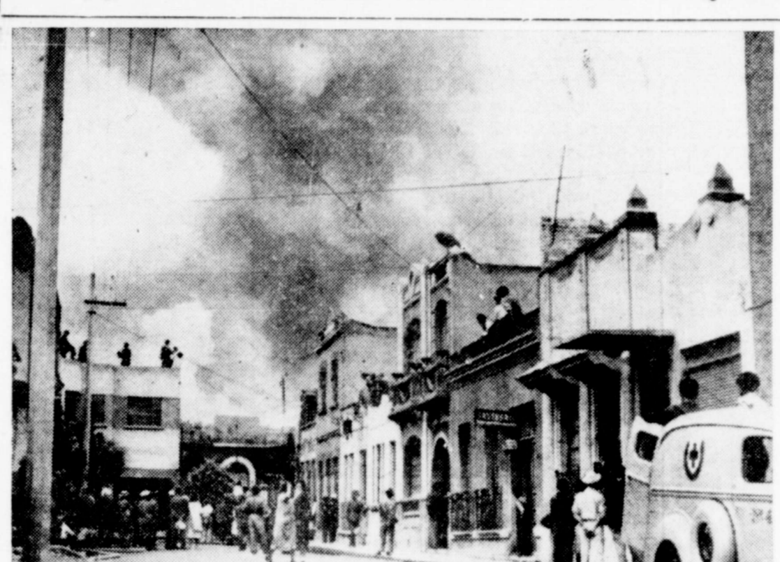
Even though the damage done was far less than in other Mexican cities, Mexico City suffered tremendous property damage in recent earthquake. Following the last tremors, an ambulance stands in Mexico City street as populace watches firemen battle flames started by the quake. (NEA Photo)
