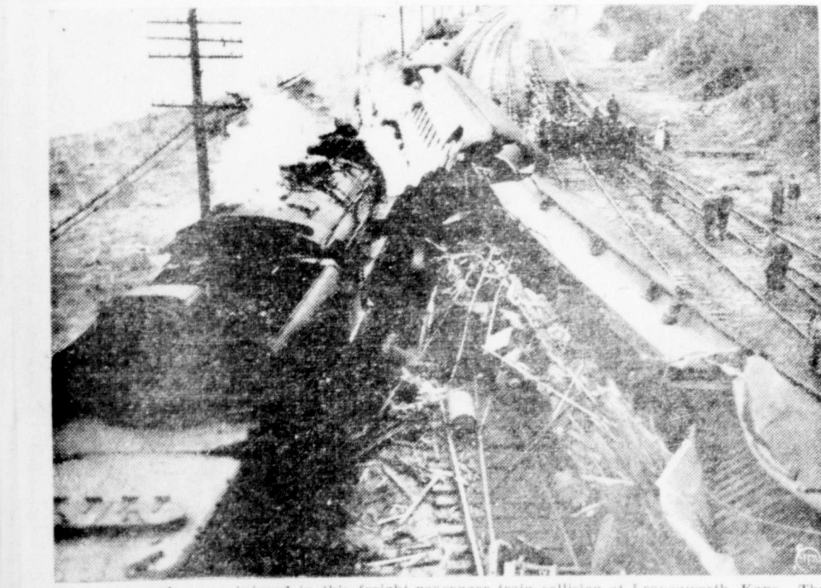
Only two people were injured in this freight-passenger train collision at Leavenworth, Kans. The cause of the accident has not been announced, but both trains apparently came together at a switch, causing the freight engine to strike the cars in such a way as to shear one side from a baggage and passenger car. (NEA Telephoto.)
