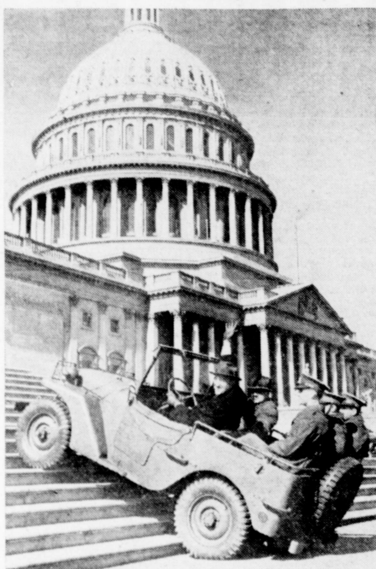
Senator James Mead of New York, at the wheel, tests army's new bantam reconnaissance car on steps of Capitol in Washington. Representative J. Parnell Thomas of New Jersey sits beside Mead. Cars weigh a ton, can make 75 miles per hour. Army claims three cars can be carried by one of its transport planes.
