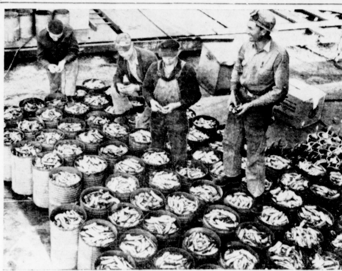
Workmen cut some of the two and a half tons of over-ripe bananas which were used to lubricate the ways for the launching of the Cape Lookout, the U. S. Maritime Commission's new freighter, which slid into the waters of the Neches river at Beaumont, Texas. Bananas provide a cheaper lubricant than grease. (NEA Telephoto)
