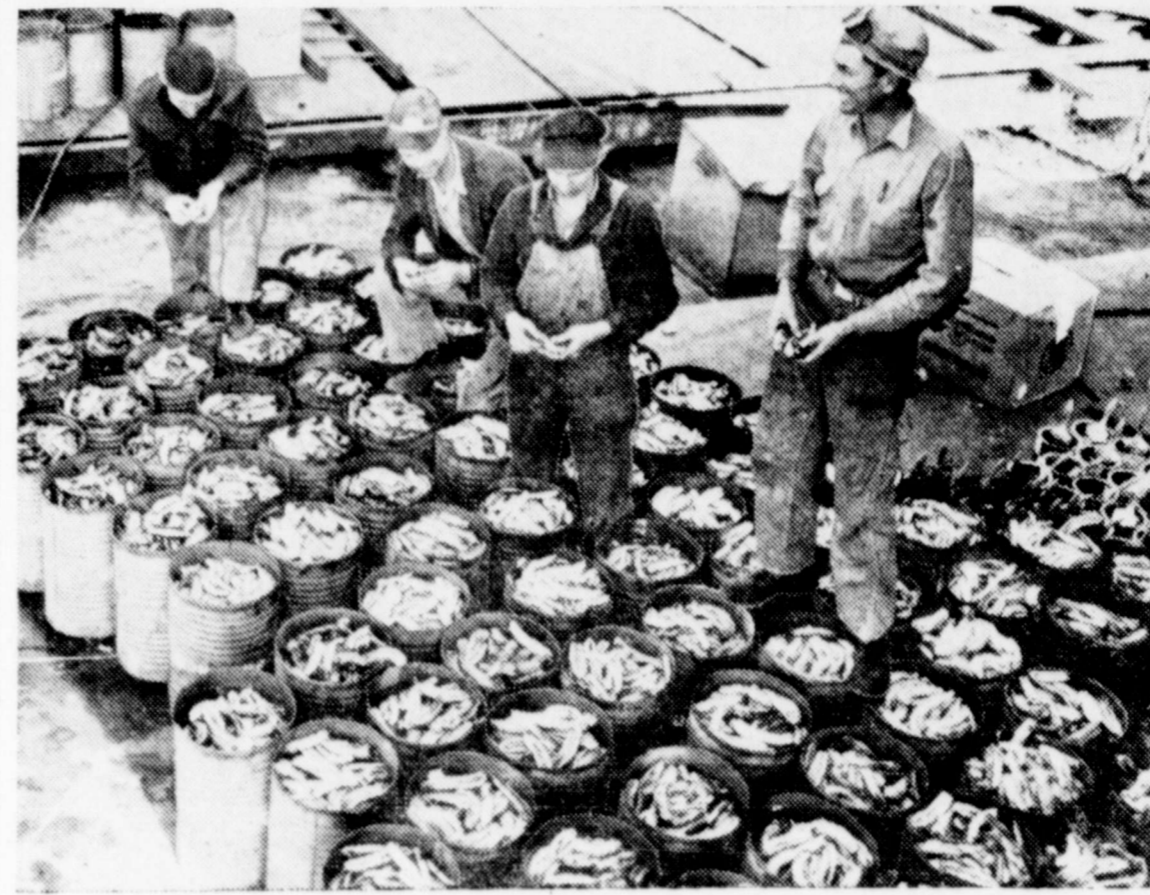
Workmen cut some of the two and a half tons of over-ripe bananas which were used to lubricate the ways for the launching of the Cape Lookout, the U. S. Maritime Commission's new freighter, which slid into the waters of the Neches river at Beaumont, Texas. Bananas provide a cheaper lubricant than grease.
