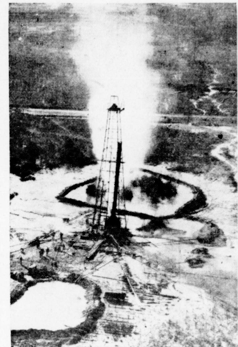
Manziel's Bell gas well near Hawkins, Texas, as it was re-opened and gas allowed to flow through the derrick to lessen danger of a crater. Later, operators pumped 3000 sacks of cement into the hole, then abandoned it. The well, which blew out of control for ten days before being checked, was reopened after gas bubbles were noted rising from ground crevices as far as 800 feet from
