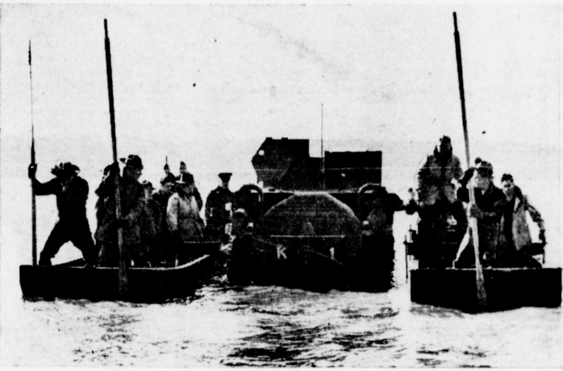
Suppose a mechanized army comes to a river, wide for quick spanning with pontoon bridges. Why, that's no problem at all, as above photo shows. In a recent demonstration of pontoon ferries, army engineers from Fort Belvoir, Va., float a medium tank across the river, supporting it with pontoons at either side.
