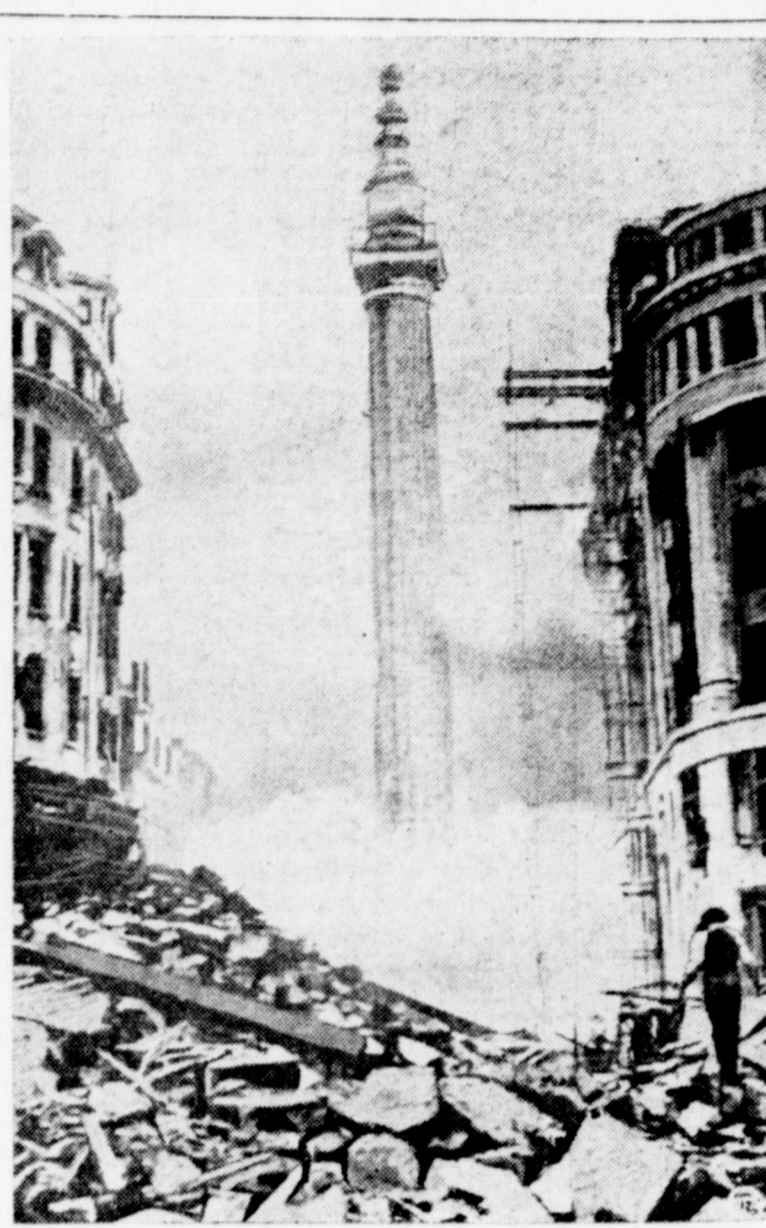
In 1666, London went through a great ordeal by fire, when a conflagration destroyed most of the city. The tall shaft in the background marks the spot where the Great Fire started. It stands amid the wreckage caused by London's current ordeal by bomb.
