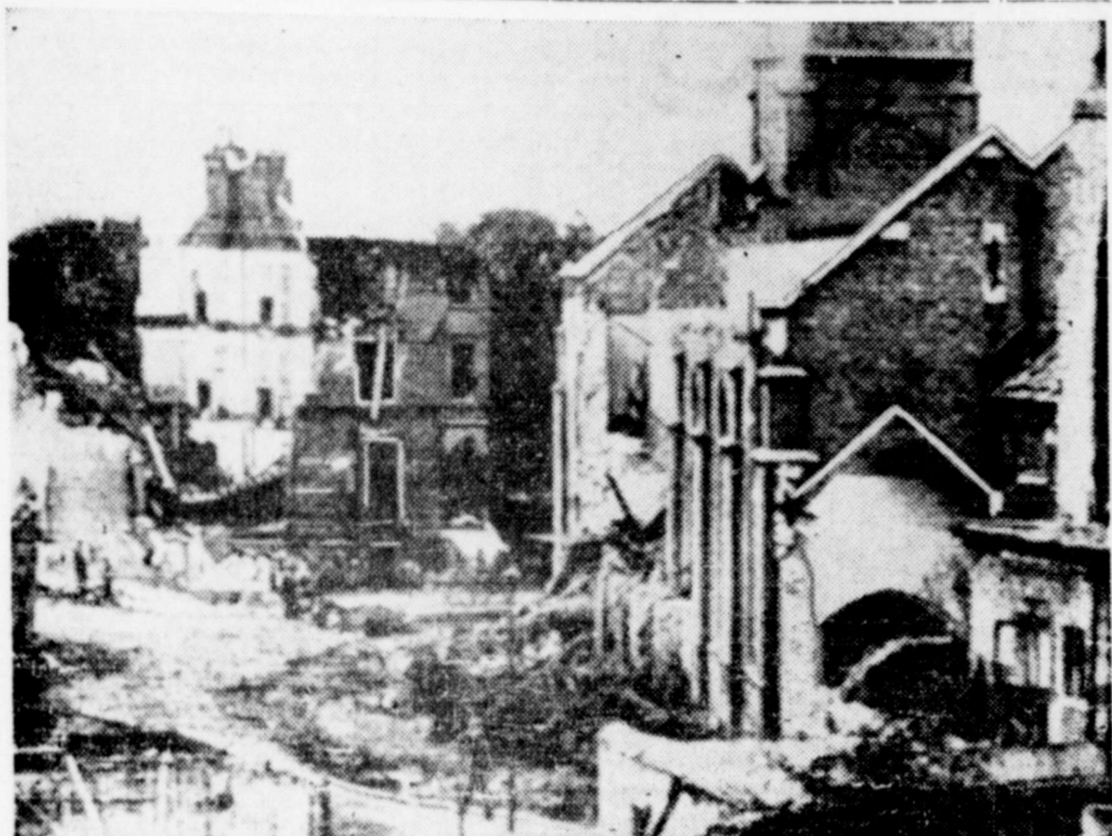
The above Cable-Telephoto gives a general view of the damage done by one German bomb in a southeast section of London. RAF fighters hurried back over the sea after wave of the Nazi ships, only a few of which escaped through the defence to drop their bomb cargoes on London.
