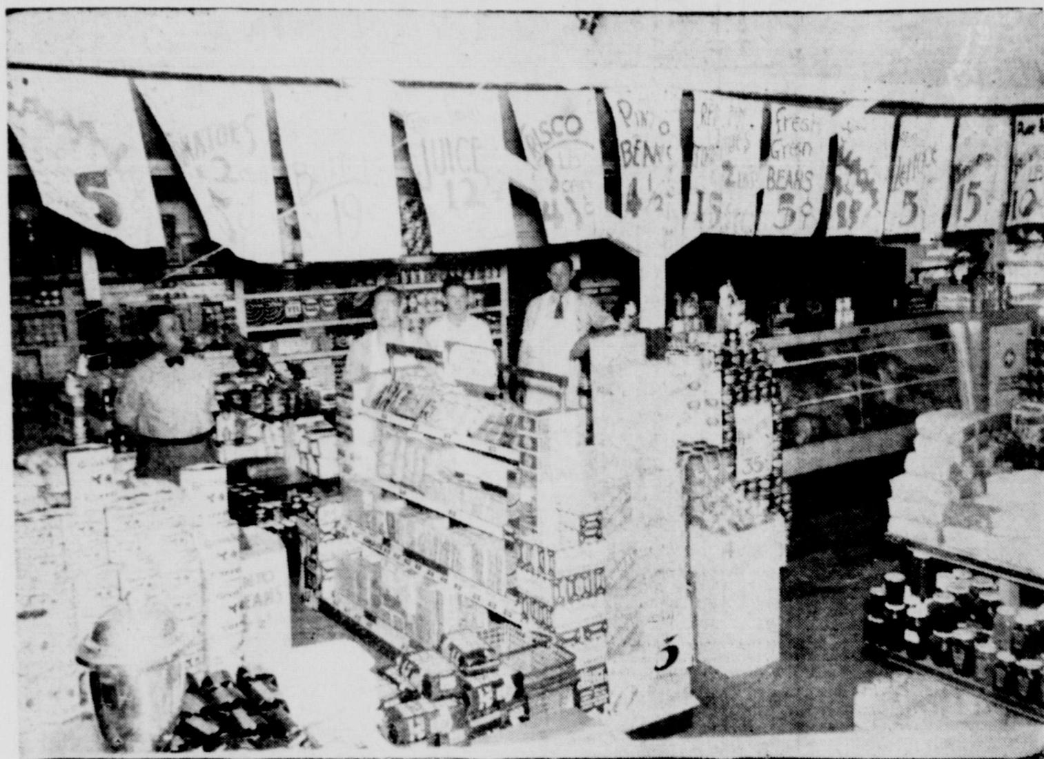
Here is an Osborn photo of the interior of the Clover Farm Grocery of Standlee McCracken and Paul Poe, recently enlarged and remodeled. In the picture, left to right, are Paul Poe, Standlee McCracken, Gale Bailey and Neal Moore.
