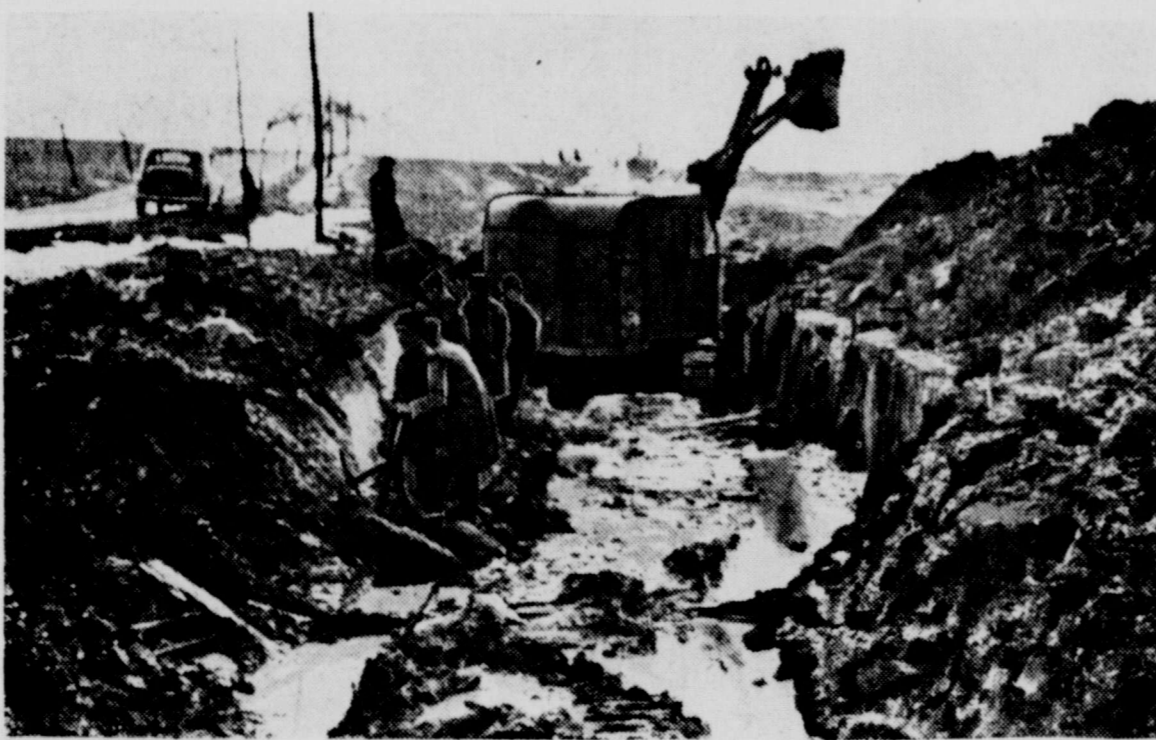
Better any day than the old hand-shoveling method of trench digging is this modern steam shovel technique, shown in use recently on the Western Front. Of course it hasn't completely replaced the pick and shovel, and the mud and water are the same as ever.
