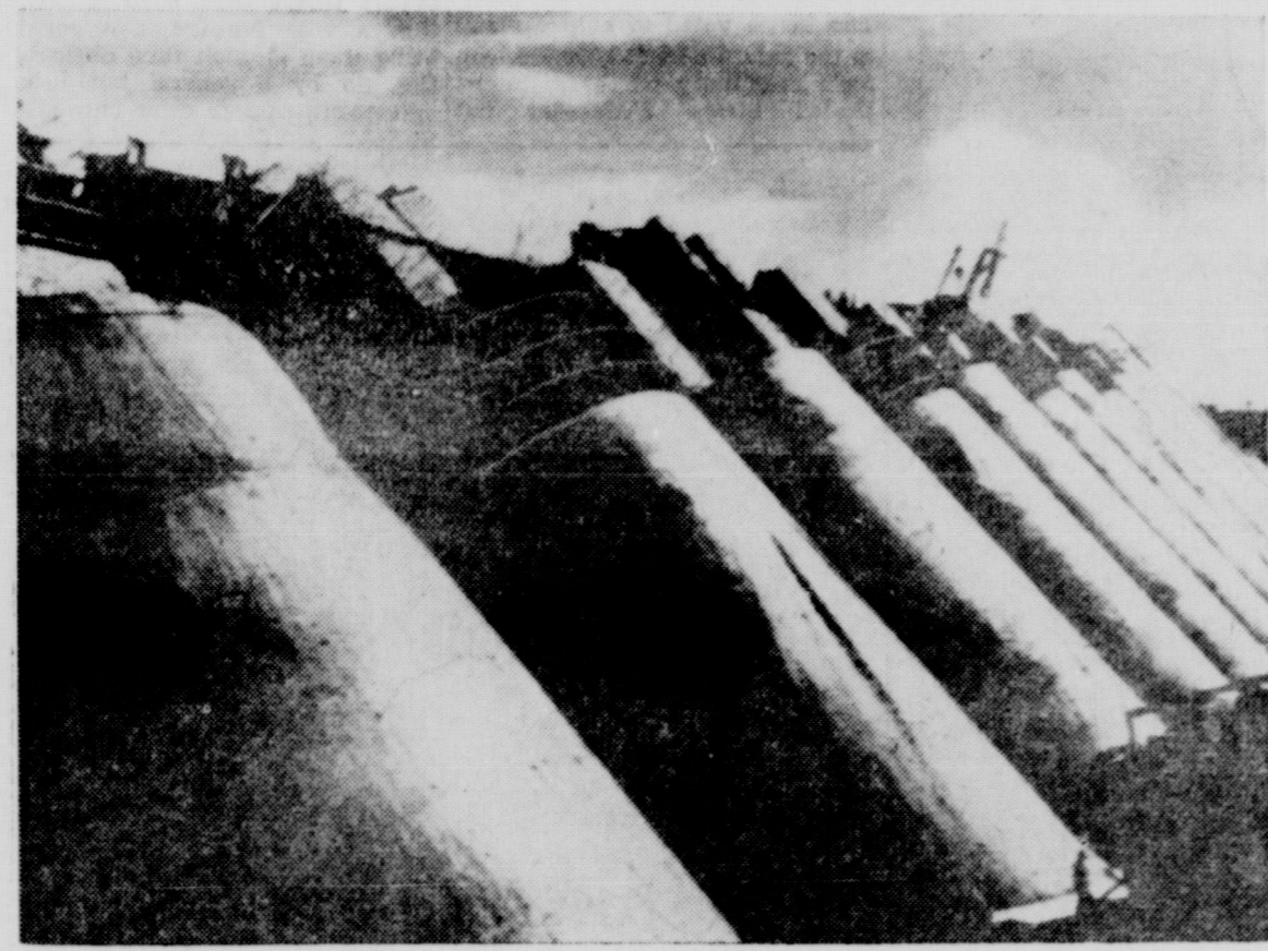
Gov. Leon Phillips of Oklahoma, will ask $940,000 indemnity from the Grand River Dam Authority for state highways to be inundated by the reservoir. He has threatened to shut-down the $20,000,000 project if the federal government does not accede. The dam is shown above.
