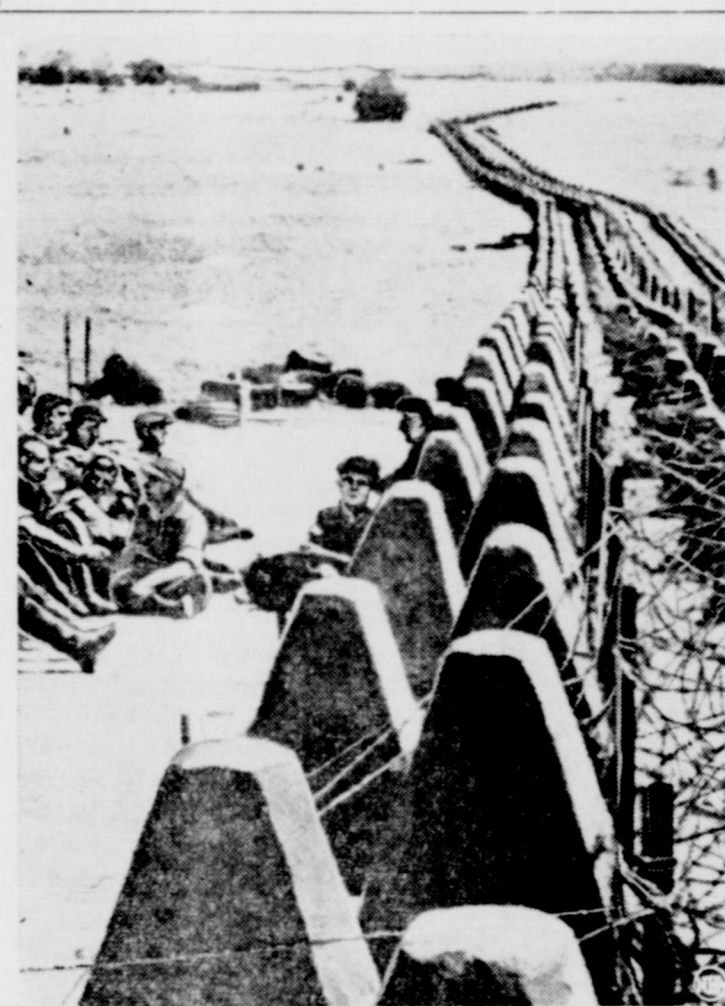
That Germany is fast becoming invulnerable against tank attack is shown in the picture, above, of concrete and barbed wire anti-tank barriers which stretch for miles opposite France's Maginot line. An important part of the new "invincible" Westwall fortifications, the barriers are being constructed by Germany's vast labor forces drawn from industry.
