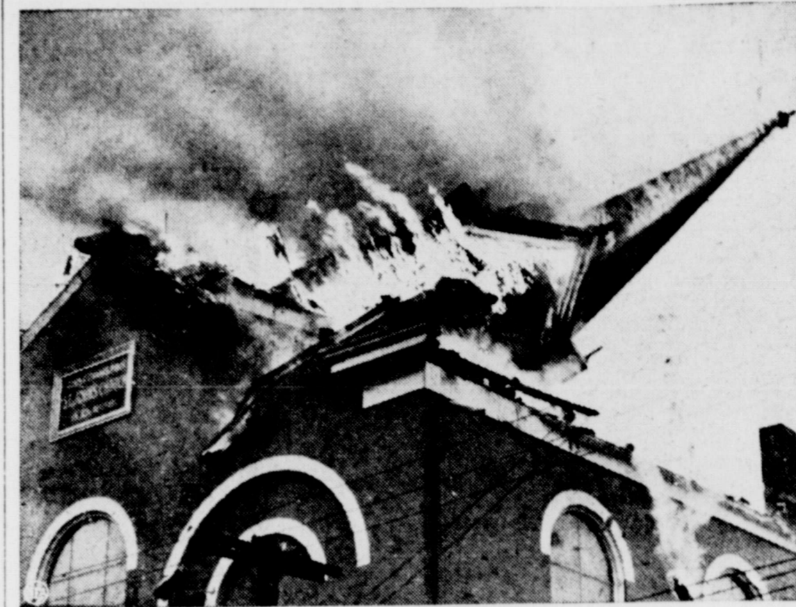
Into the church interior crashes the flaming steeple of venerable St. John's Evangelical Protestant Church at Newport, Ky. Damage was estimated at $75,000.
