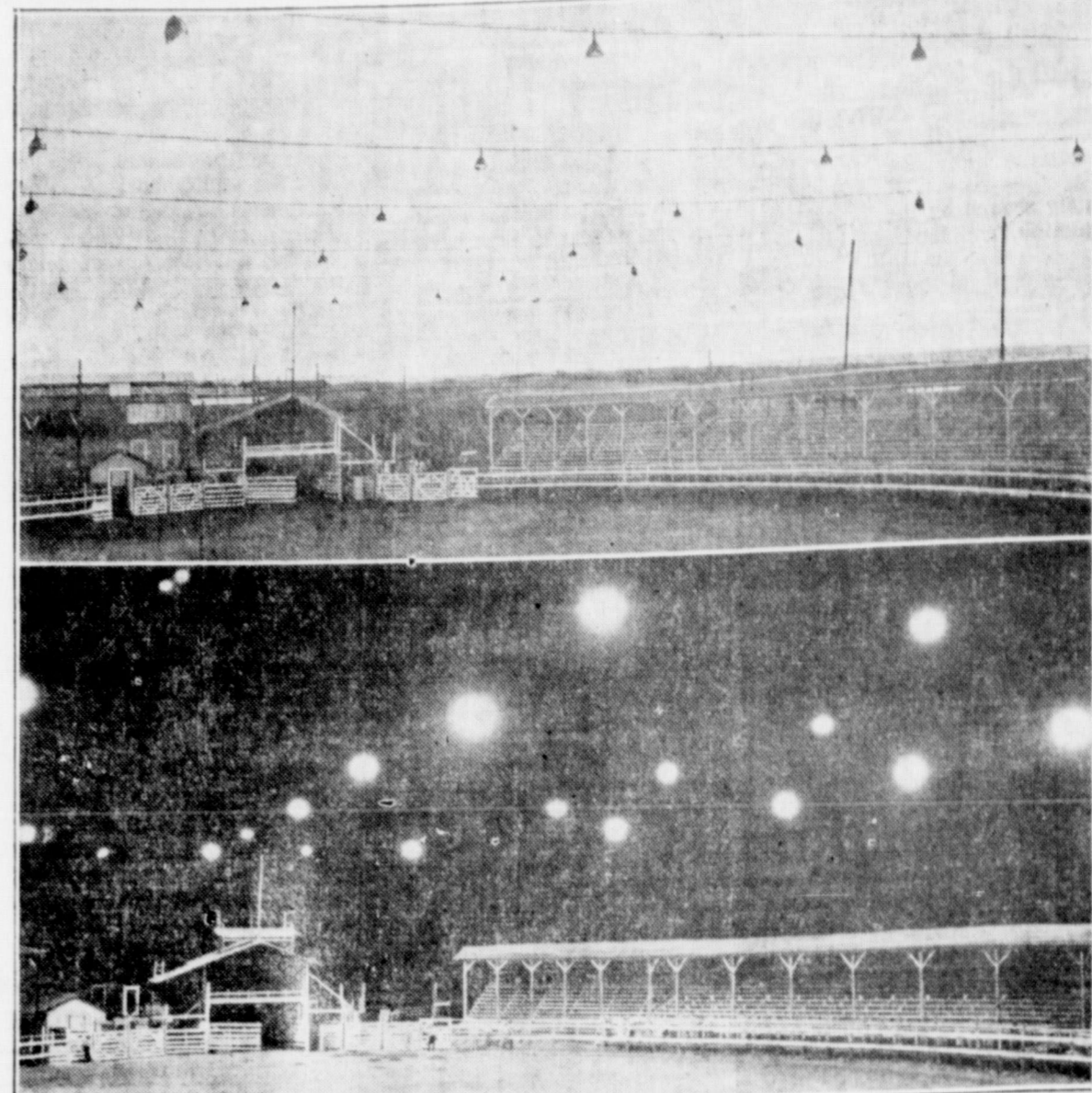
Eight times as much light as in previous years will beam upon rodeo performers in the arena of the Texas Cowboy Reunion at Stamford July 1-2-3. Above is a daylight view of the arena in contrast to the lighted scene by night (below) when cowboys will "do their stuff" under 26 overhead lighting units of 1,500 watts each—just installed by the West Texas Utilities Company. Eighteen lighting units of 1,500 watts each light up the Reunion grounds.
