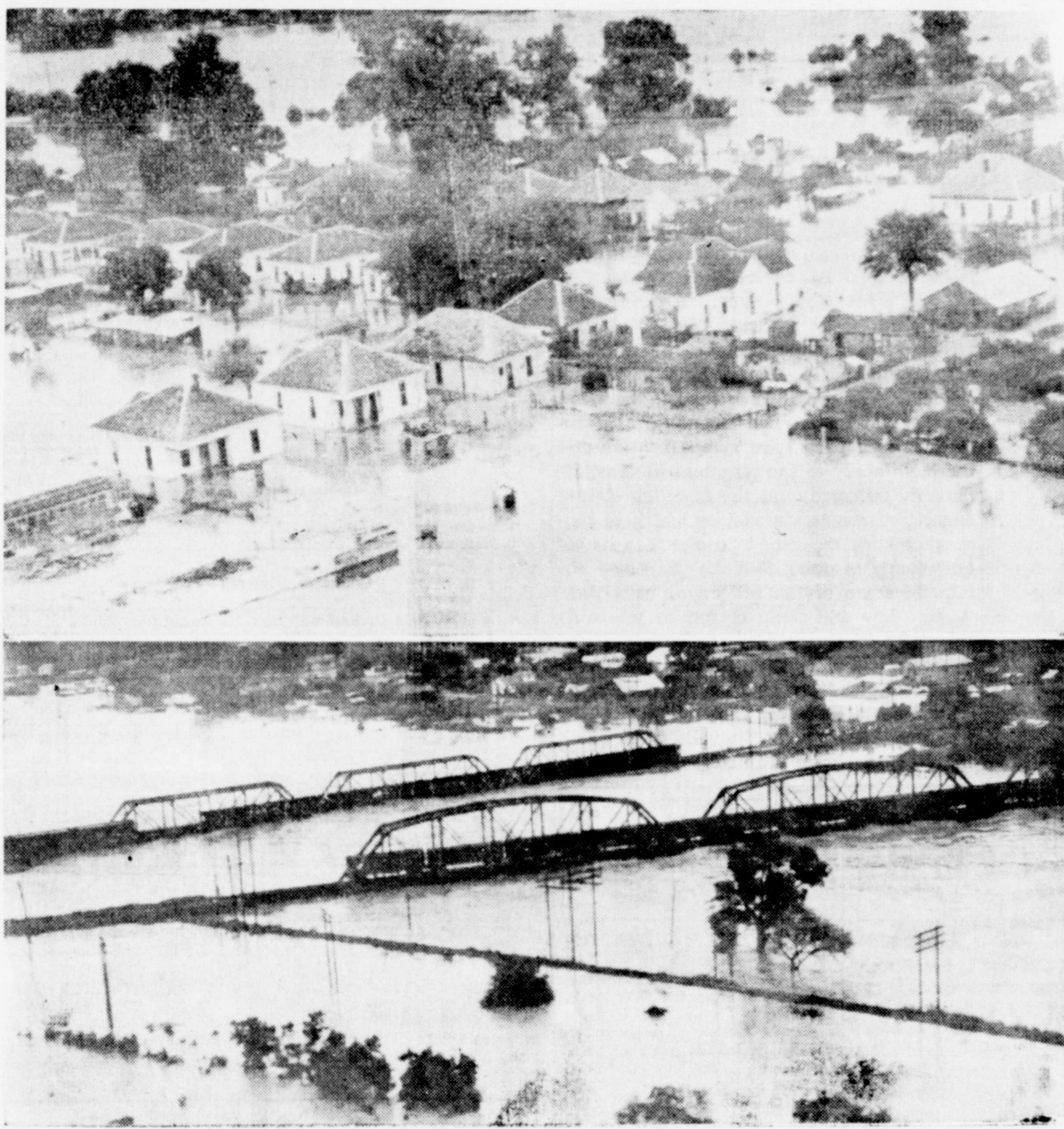
Two thousand persons were homeless when the rampaging Brazos river broke through its levees and flooded East Waco's residential and industrial area. The photos above show: Top, part of the residential section as the water was ascending. Bottom, two railroad bridges, strengthened with strings of freight cars hastily rolled out to furnish added weight against the push of the flood and debris. (Associated-Press Photos)
