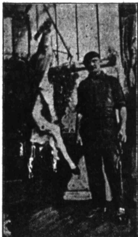
A Slaughterhouse Where Inspection Is Not Maintained.
