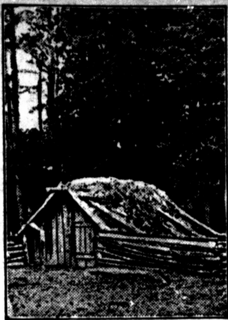
An Outdoor Storage Cellar, Typical of Those Used in the South for Storing Sweet Potatoes and Other Root Crops. It Consists of a Pole and Plank Frame Covered With Sod and Straw.
