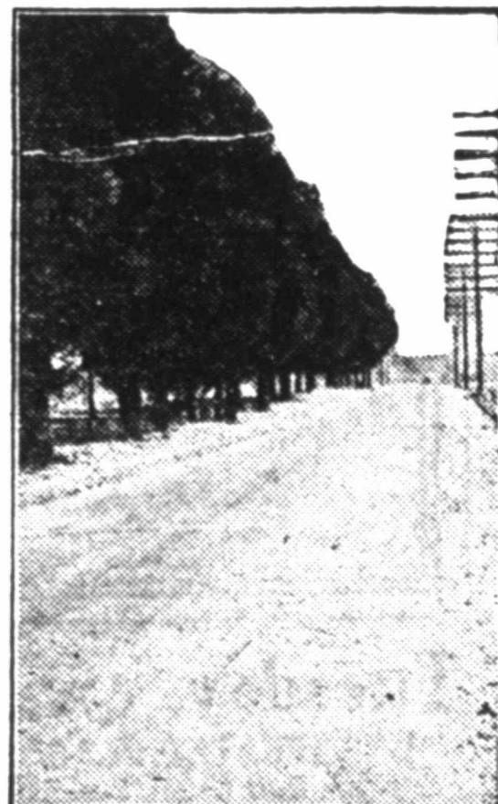
Good Roads Between Annapolis and Baltimore—Job for Many Men to Build and Maintain Road Like This.
