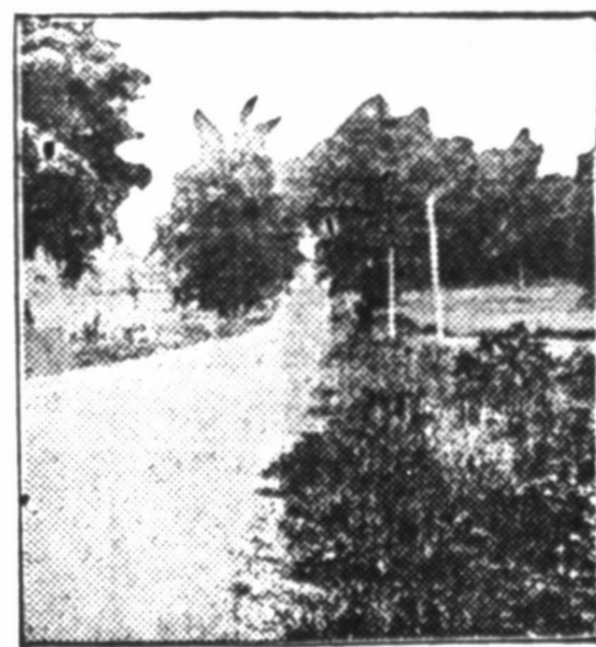
Bituminous Macadam Road.
