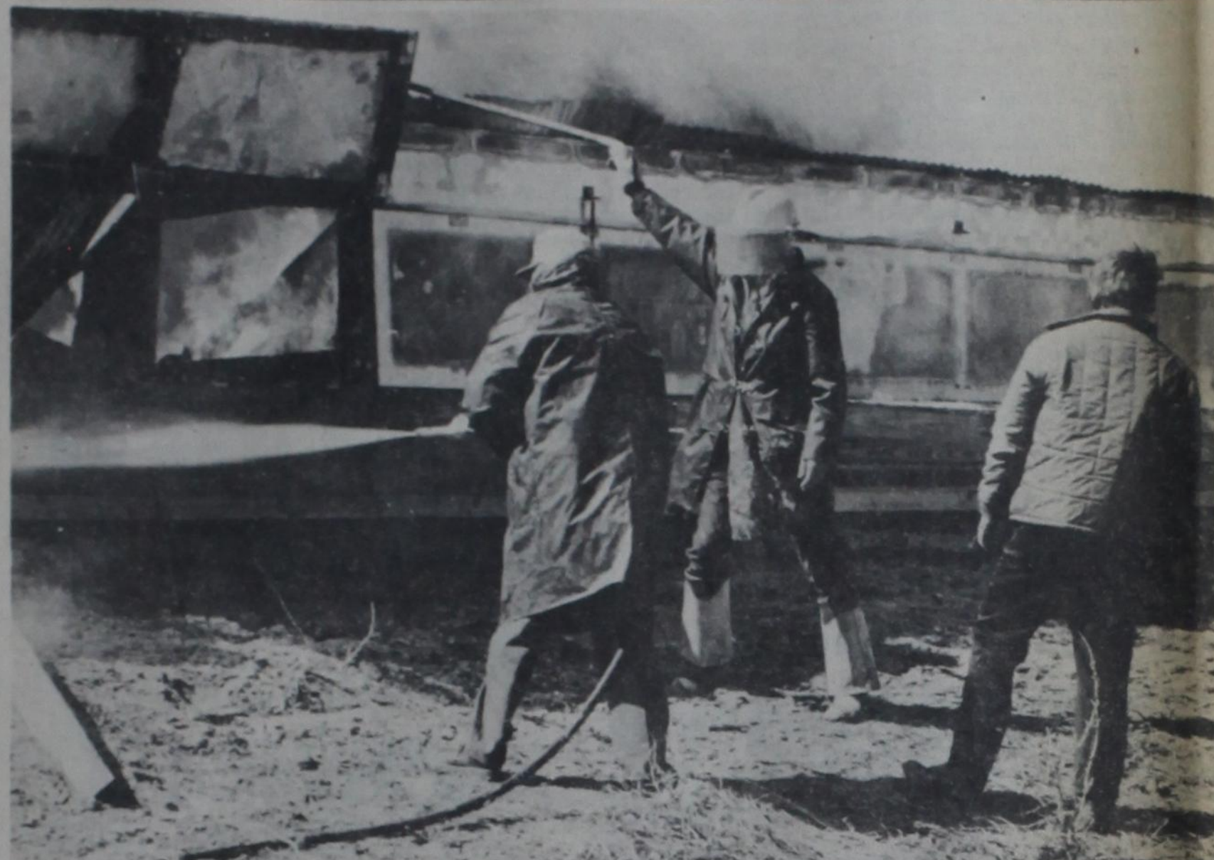
HEAVY DAMAGE resulted from this fire last Wednesday at High Plains Park, seven miles west of Dimmitt. Despite the efforts of Dimmitt volunteer firemen, this hog barn was virtually destroyed by wind-whipped flames, although the fire was kept away from other buildings. Fortunately, there were no animals in the barn. Fred Bruegel Jr., owner of the SPF hog operation, estimated a 75% loss on the building.
