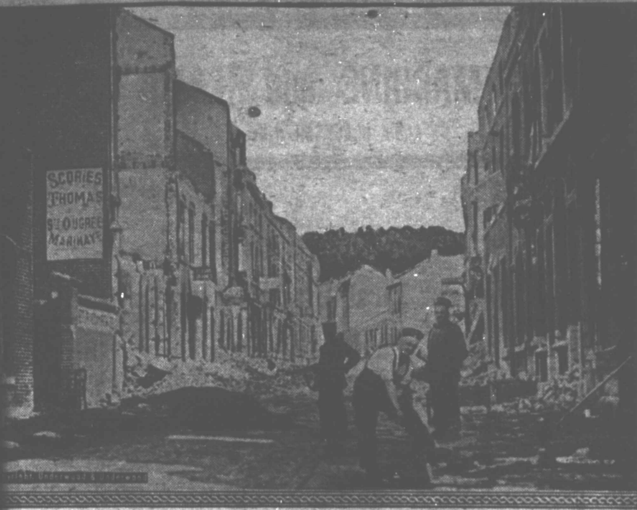
Because Yise, Belgium, offered a stout resistance to the German troops they left it in the condition here shown, a mass of ruins.
