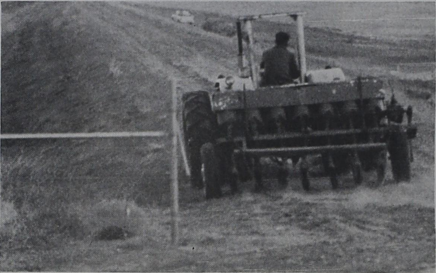
The flood control dam, east of Sunnyside was re-planted in grass this year. The dam area has not formed a good grass cover to protect it. The spillways have a good stand of grass and didn't need re-planting. The site was planted to a mixture of 5 different grass species.
