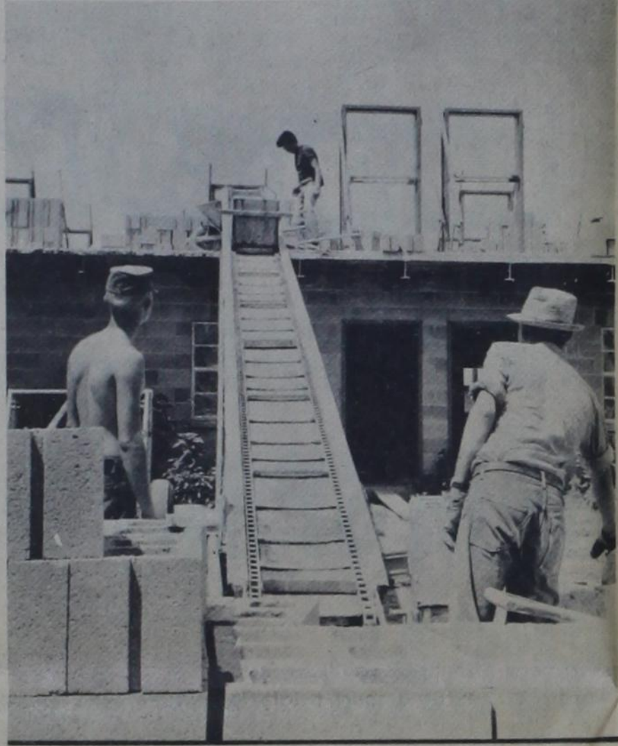
UP GOES THE MORTAR, sent via mechanical mule by Ken Campbell and Gary Jennings, to Joe Flores on the second story level of an MHP apartment building. The project called for the biggest single concrete-block order in West Texas history.
