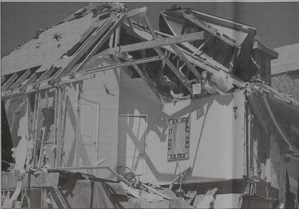
Houses along Panhandle Street, in the Dalton Ranch subdivision were destroyed, during the early morning hours of March 29, 2017, due to severe storms. The National Weather Service concluded the damage was caused by straight-line winds.
