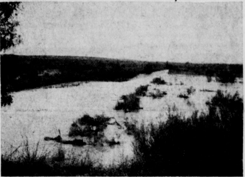
Brush Hangs at Top of Spillway, Water Goes on Over
