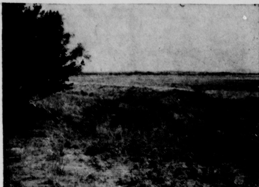
LEVEL SPILL — This diversion terrace in the background drains into a level spill in the center of the picture. The level spill drains into a pond on the right. Note the good cover of grass and no erosion. These structures are located on the Robert Hickman Ranch.
