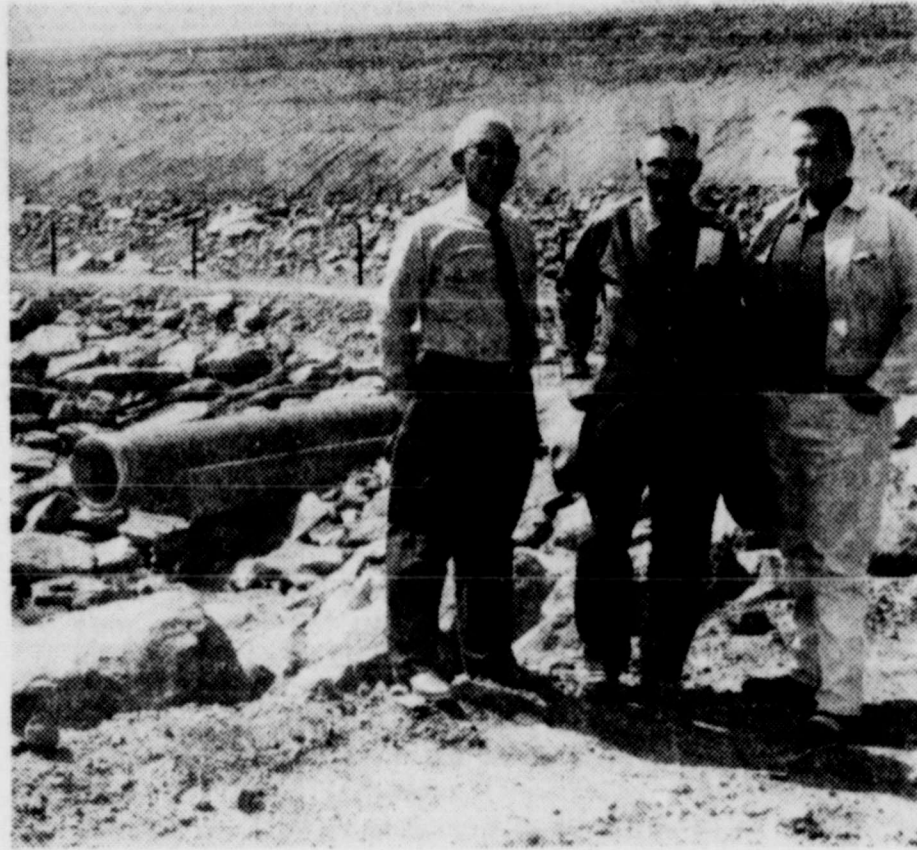
W. E. Burns, Robert Walker, ranchmen, and J. R. Haralson, Robert Lee, with the Soil Conservation Service, were looking over the completed dam on W. D. McDonald land when the photographer came along. In the background is the "draw down" pipe, which will let the water out of the lake down to 200 acre feet, which water is kept for the use of the landowner who furnishes the land on which the structure is built.
