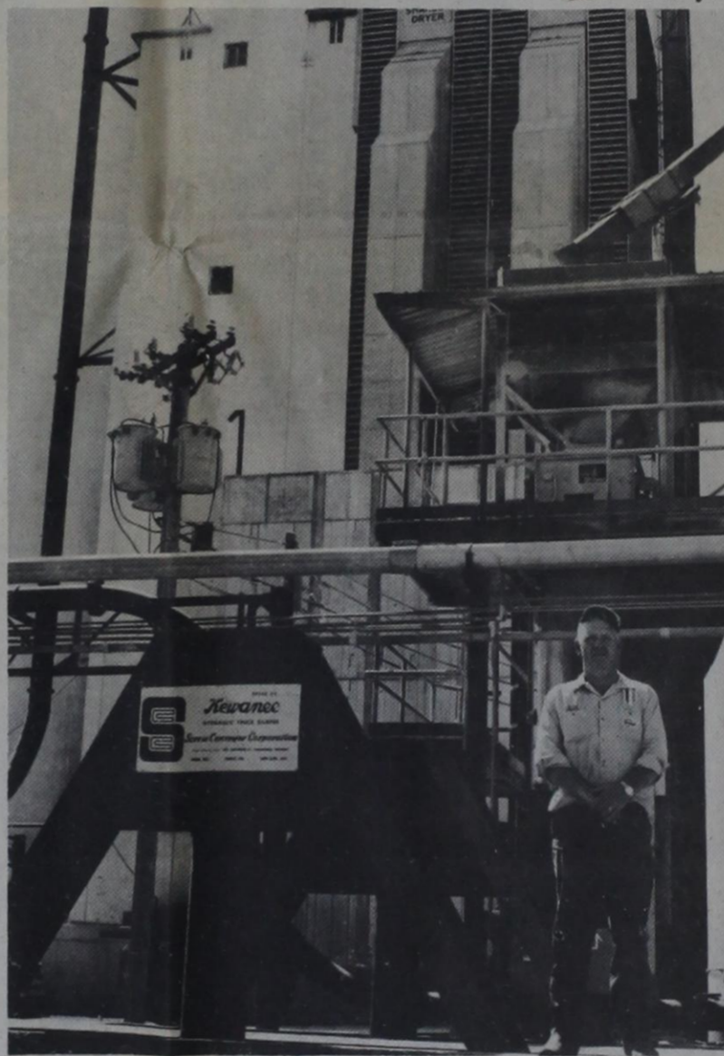
AN ADDED SERVICE at Dimmitt Agri Industries, Inc., this year is the new "semi dump" for tractor-trailer rigs. Here, Elevator Supt. Bill Goldsmith stands alongside the new Kewanee hydraulic truck dumper. In background is the world's largest corn dryer.
