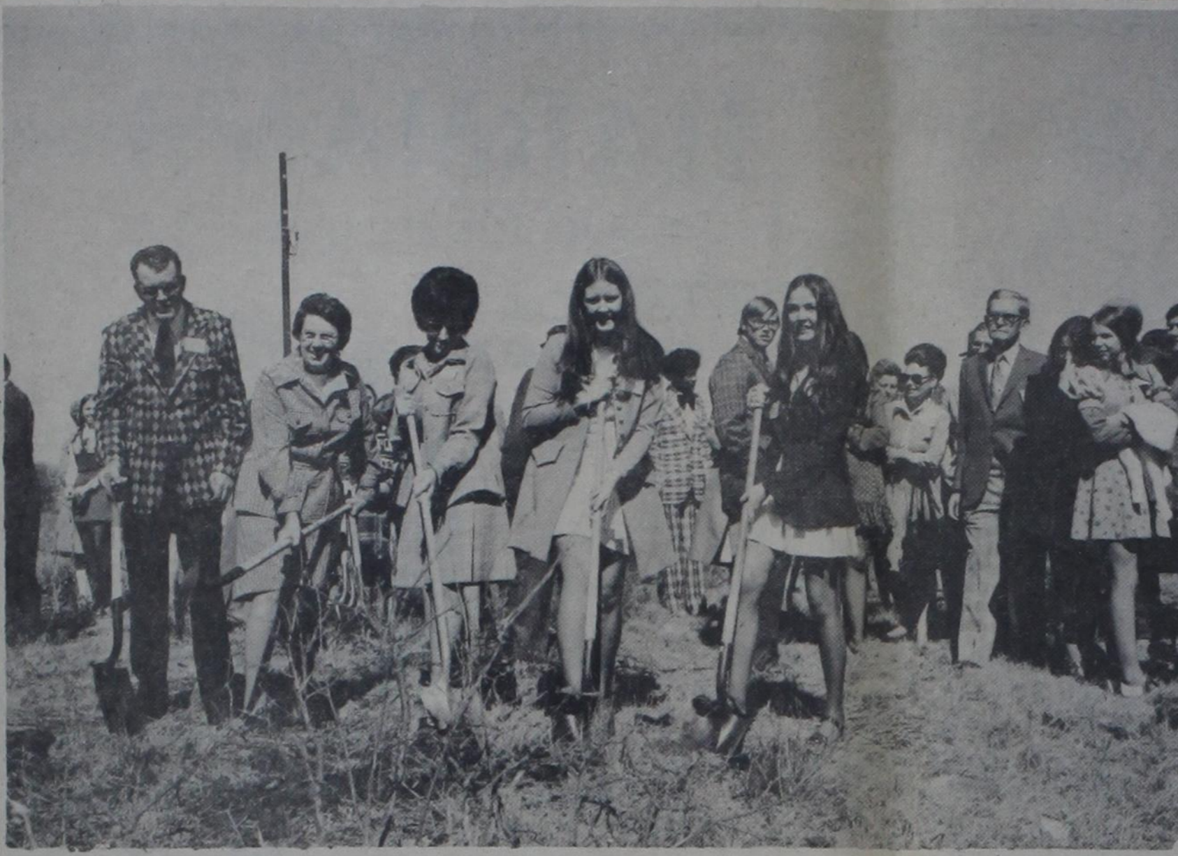
CONSTRUCTION ON TEXAS' new $1.375 million 4-H Center is getting underway on a scenic 78-acre site overlooking Lake Brownwood. Present at the groundbreaking ceremony at the lake site was this delegation from Extension Service District I. Pictured left to right are Mr. and Mrs. Jack Ingram of Dimmitt,
