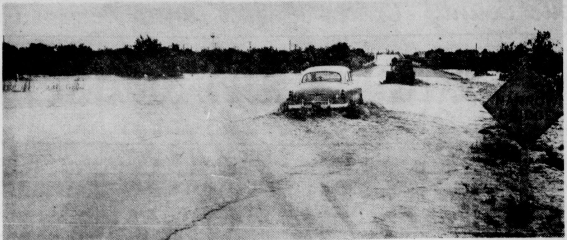
COLORADO RIVER GOES ON RAMPAGE —Overflow waters from the Colorado River, sweeping around the south end of the Robert Lee Bridge, fell just short of blocking traffic there at mid-
