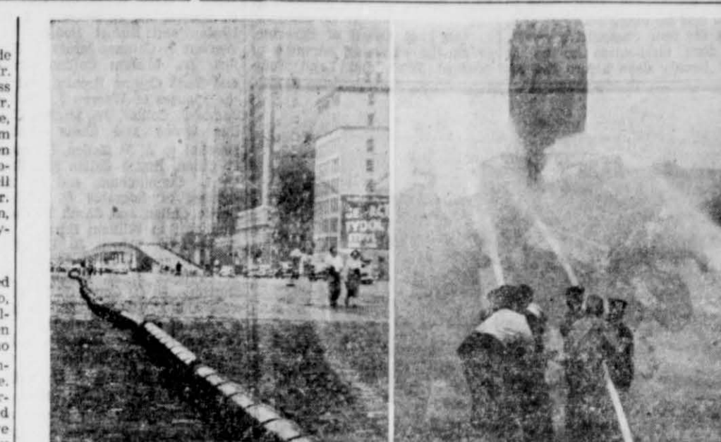
DEMONSTRATION OF FIRE in New York City which can be laid quickly over rough terrain to carry water for fire fighting, city water supply lines allow pipe to be laid without leveling it.
