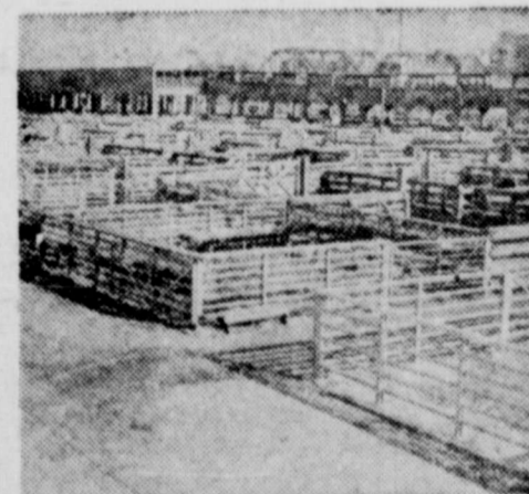
The Chicago Stock Yards, which marked its 85th year on Christmas day, 1950, moves ahead toward better service for the livestock farmer. Here is shown a row of galvanized steel pens that are replacing the old wooden pens at the yards. They are fire-proof, rust-resistant and their smooth edges prevent bruising of cattle.
