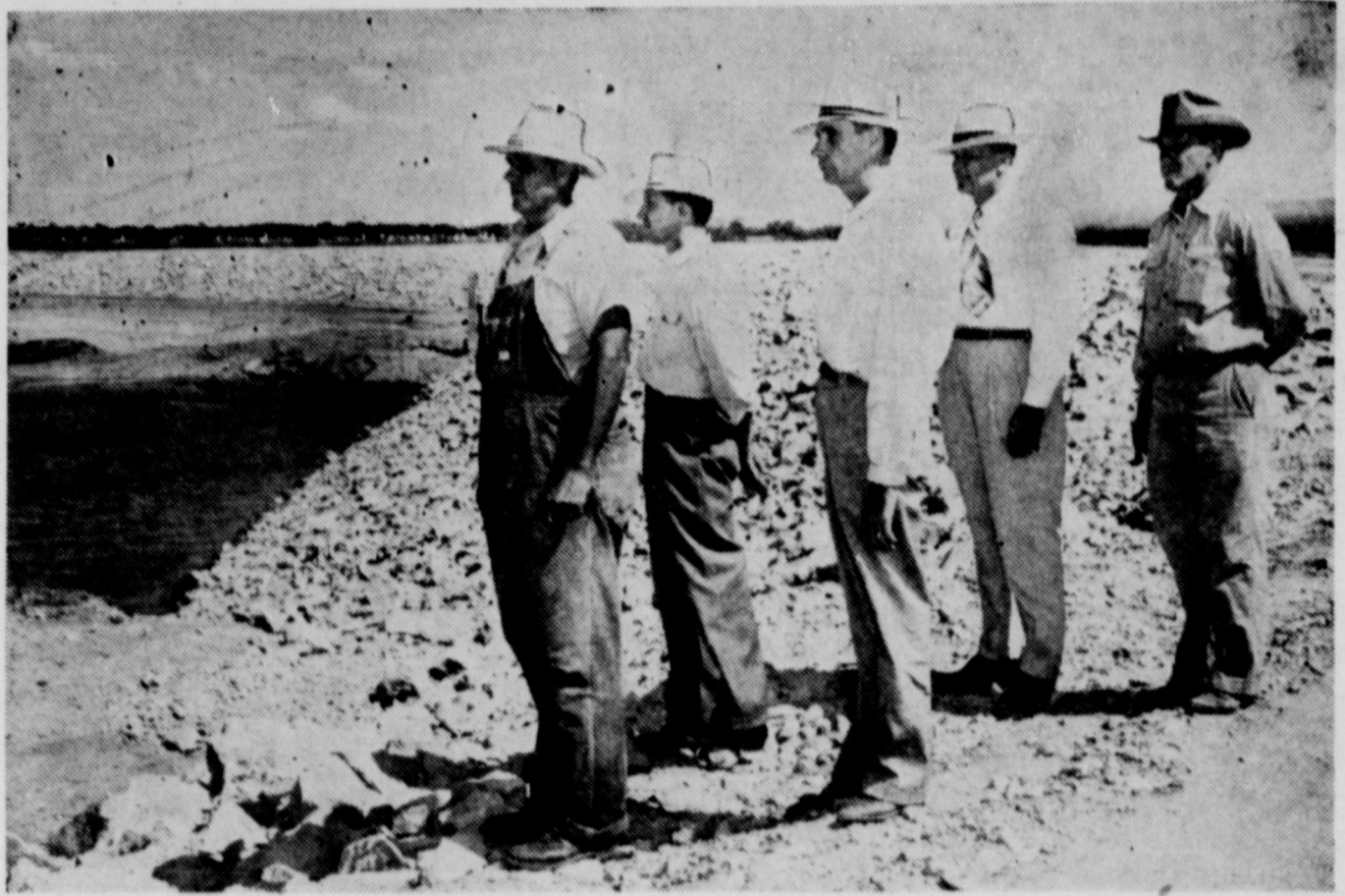
'READY FOR A FLOOD' —The Upper Colorado River Authority-financed Robert Lee dam on Mountain Creek here stands finished, ready for a filling deluge. Standing on top of the dam looking toward the embryonic municipal supply lake are Water Supt. Sam Jay, UCRA Director Cumbie Ivey, J. A. Roberson (his firm held the $62,727.50 construction contract). UCRA Secretary Gerald C. Allen and City Commissioner Fern Havins
