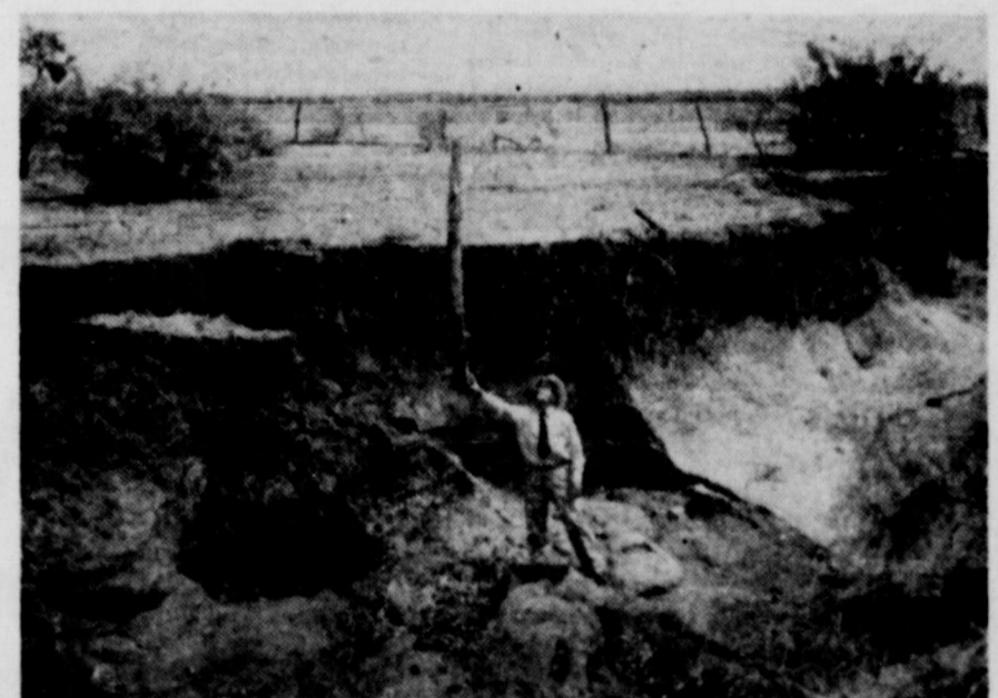
Uncontrolled road water caused this erosion damage in the Green Mountain community. E. J. Hughes, District Conservationist with the Soil Conservation Service, measures the depth of the cut. The Coke County SCD is working jointly with the County Commissioners Court, the Texas Highway Department and the land owners in correcting this problem of community concern.
