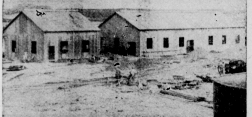
BOILER BUILDING (L) and generator building.
