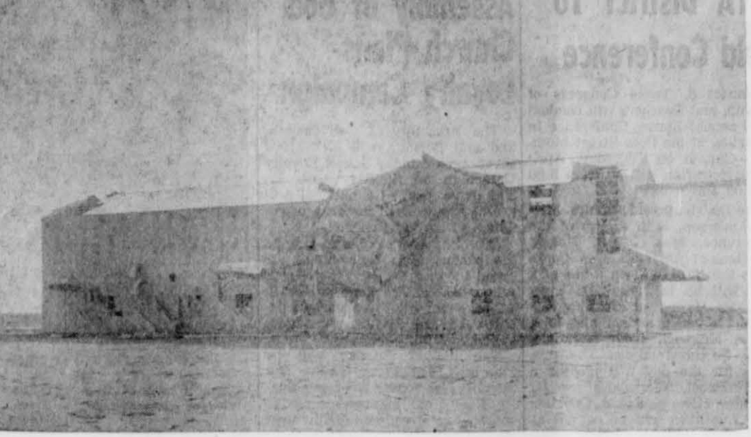
GIN DAMAGED—Heavy damage resulted to the Hogan Gin in Tuesday night's tornado which hit Sunnyside. The owner, T. R. Hogan, was killed in the vicious wind. Completely demolished was the unloading shed on the west side of the gin.
