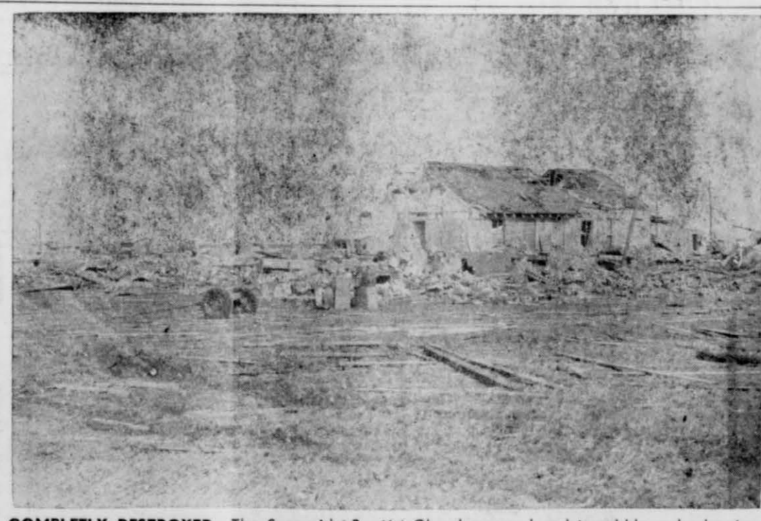
COMPLETELY DESTROYED—The Sunnyside Baptist Church was reduced to rubble and a leaning, sagging frame portion Tuesday night following a tornado that hit about 8 o'clock. The concrete block structure, the part that blew down, was almost new. There were about 135 people eating supper in the old part when the first warning was sounded.
