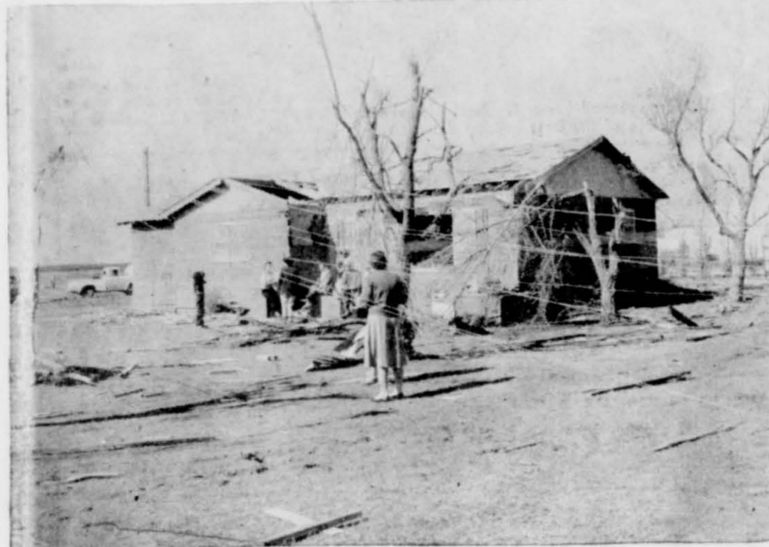
THE AFTERMATH—These residents of Sunnyside study the damage and ponder their respective situations Wednesday morning following the tornado Tuesday night which almost wiped out the small community.
